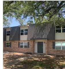
RENAISSANCE OAKS HOUMA IN CONSTRUCTION
