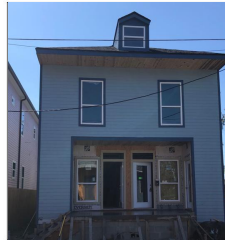
NORA St. ANN, NEW ORLEANS IN CONSTRUCTION
