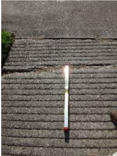
Curb ramp west side of crossing from Center to B1.
